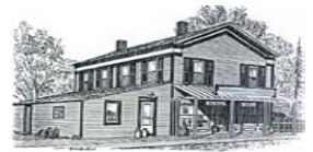
Mercantile Building and Information Center 1856
